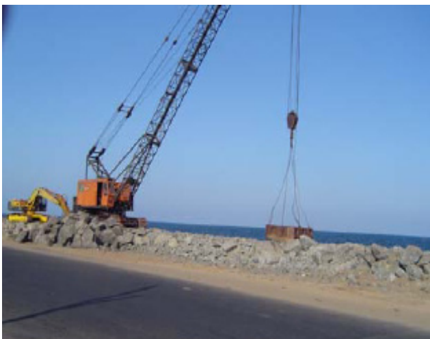
Rubble Mount Seawall under construction.
