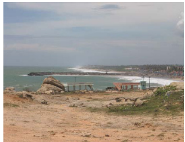
Pre-tsunami breakwater: Kovalam, Kanyakumari district.
