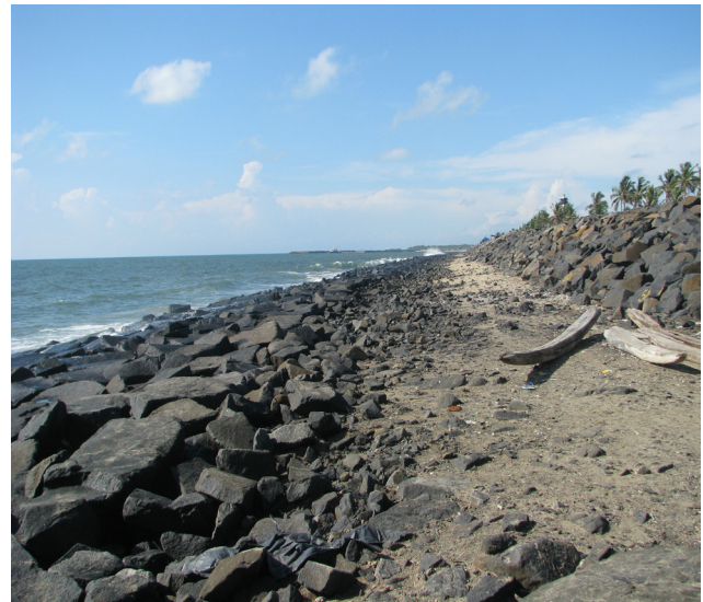
Seawall construction on the beach affects sand dynamics of the beach and in turn affects sand budget of coastal dunes.
