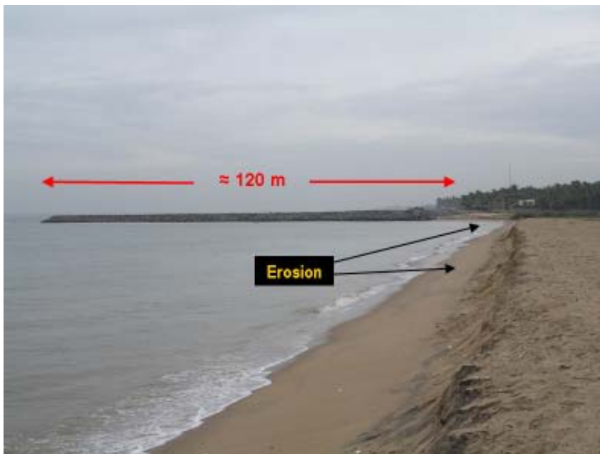
Groyne built North of Thandirayankuppam Village in Tamil Nadu May 2007
